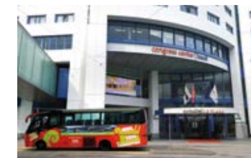
08 Swissôtel / Messe Stops in front of "Swissôtel Le Plaza", main entrance 📍 Messeplatz 25
